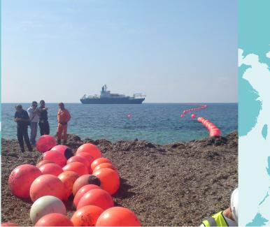
Tunisie Telecom contracted (Huawei Marine Networks) HMN and Global Marine Systems Limited for the supply and installation of fibre optic cable for the Hannibal submarine cable system between beach manholes in Kelibia, Tunisia and Mazara del Vallo, Sicily. The 177.5 kilometres of submarine cable was provided by Nexans, and loaded at the port of Rognan, Norway.
